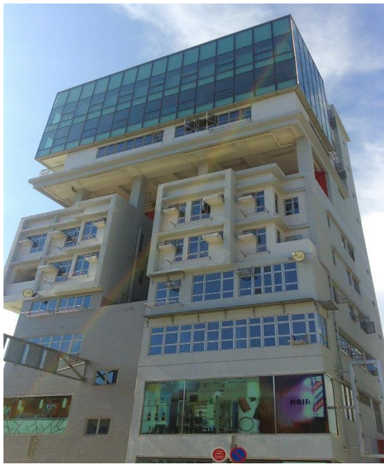
Rescue Training Tower
